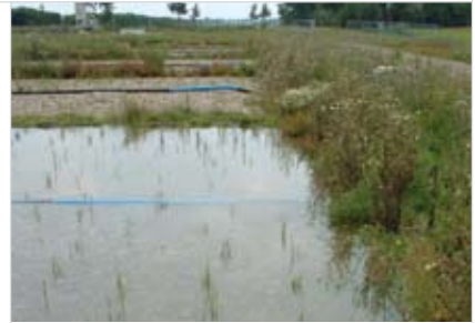
The vertical flow system of reed beds was highly successful in reducing phosphates and pathogenic bacteria
