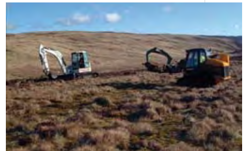
Blocking ditches restored the bog water level
