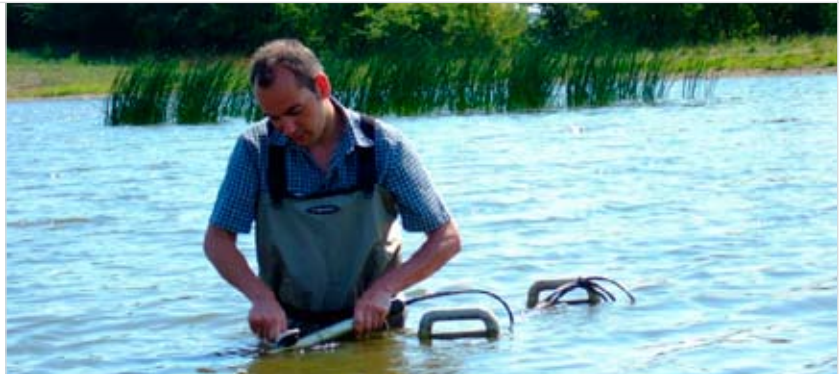
A wet retention pond with a sand filter and fixed-media absorption filter was used to remove pollutants from urban run-off water
