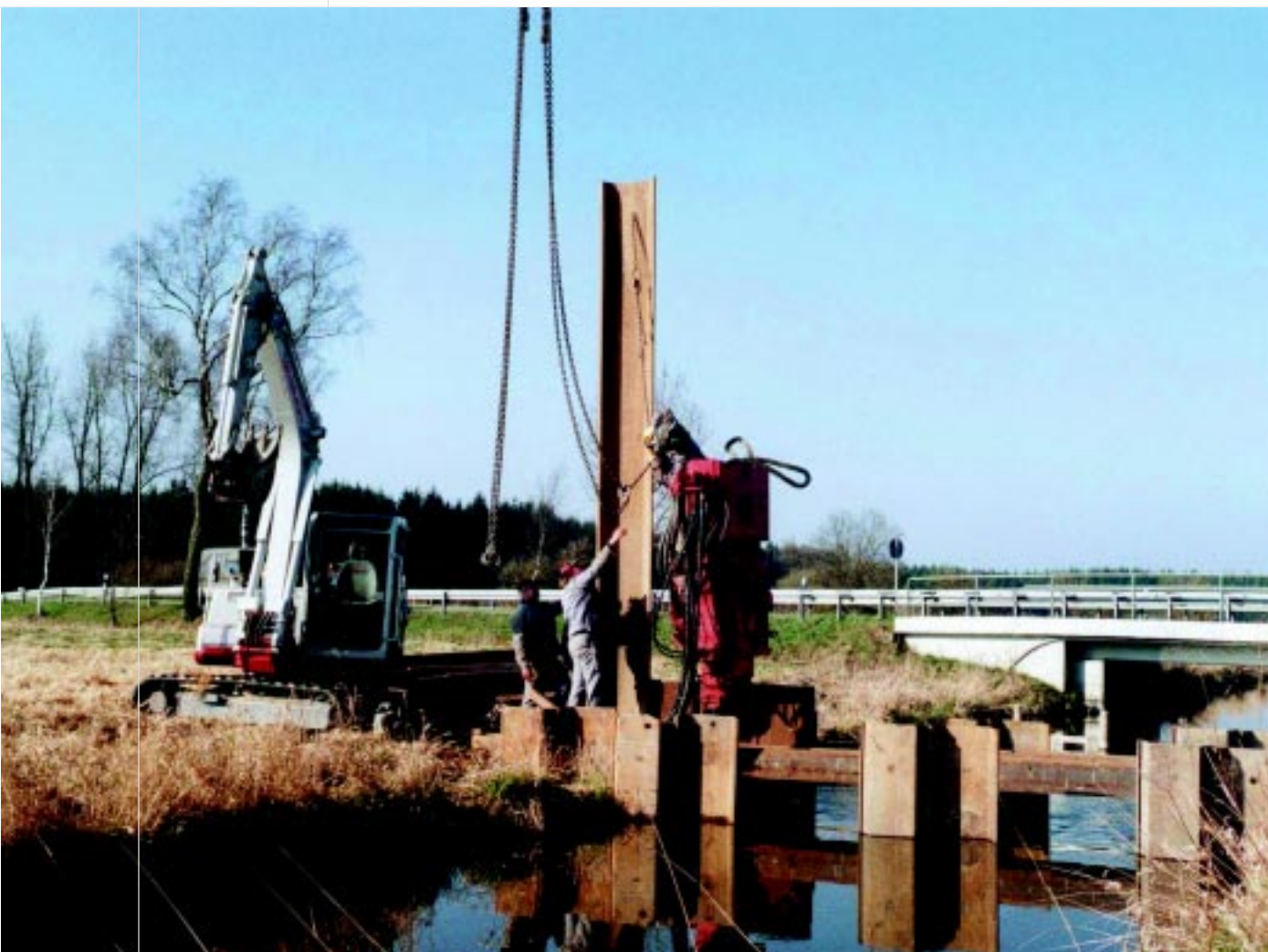
Building a dam across the Kanzach stream to raise water levels. (LIFE project "Federsee"). Photo © Jost Einstein
