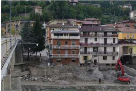
Figure 1: Bridge at Farini along the Nure river after the event of the 13<sup>a</sup> - 14<sup>a</sup> September. The river entered the ground and first floor of the houses, reaching an hydrological level of 7m observed by
